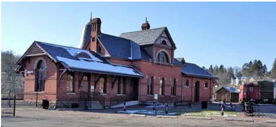
Oakland Maryland B&O Railroad Station – street side
