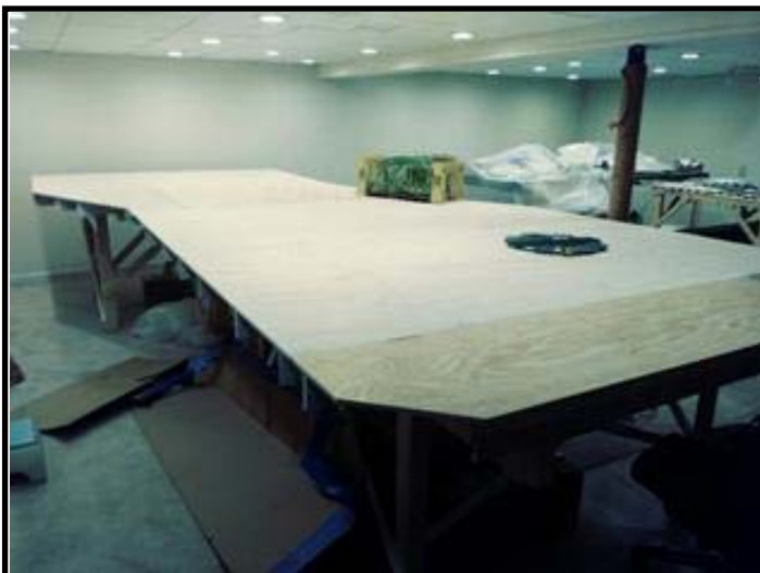
Finished benchwork. Note the 30-degree transition mid-layout.
