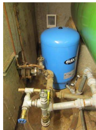
High Zone pump and hydro-pneumatic tank in the High Zone pump station basement.
