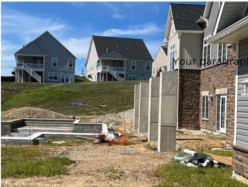
Support pillars for the sun deck in place
