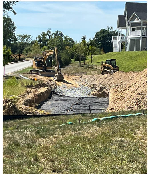
Leveling the basin behind the clubhouse for proper runoff
