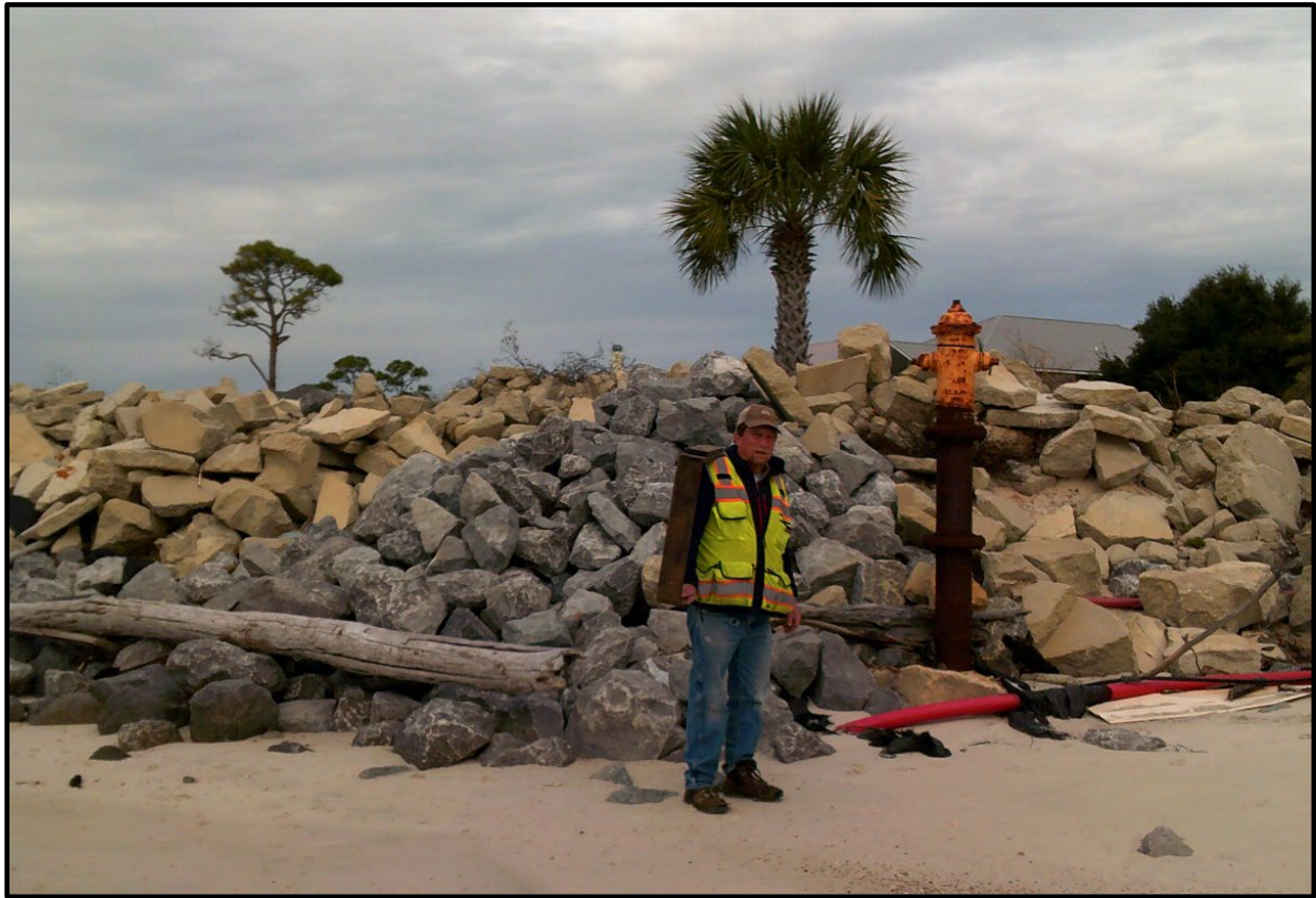
Figure 23. Western limit of project area. Fire hydrant indicates the amount of shoreline lost since 2016.
