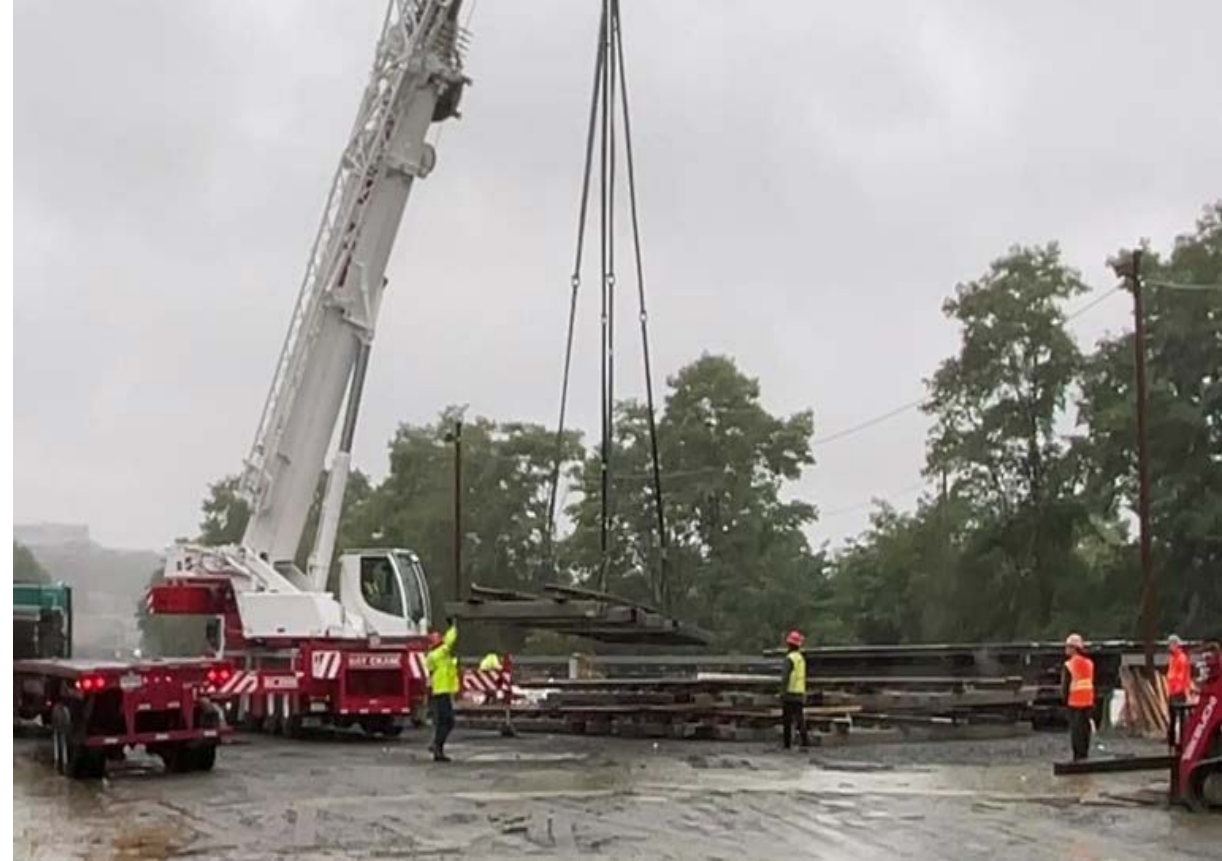
Delivery of Leggett Crossover special track work
