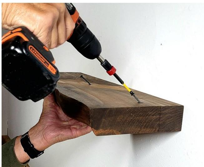
**Step 3:** Once the rear section has been mounted, slide the front section of the shelf over the dowels tight back against the rear piece. Lastly, fully insert the shorter 2" screws into the predrilled angled holes on top of the shelf.
