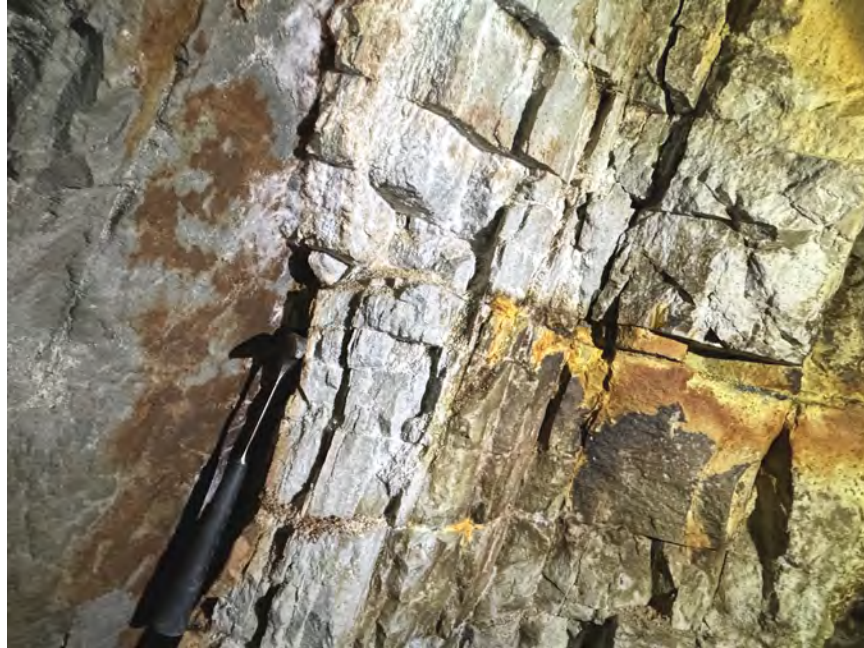
Figure 24: Close-up of above; fractures in the altered latite dyke are well-developed, some of which are mineralized, but the limestone is neither fractured nor mineralized, lower Arrance workings
