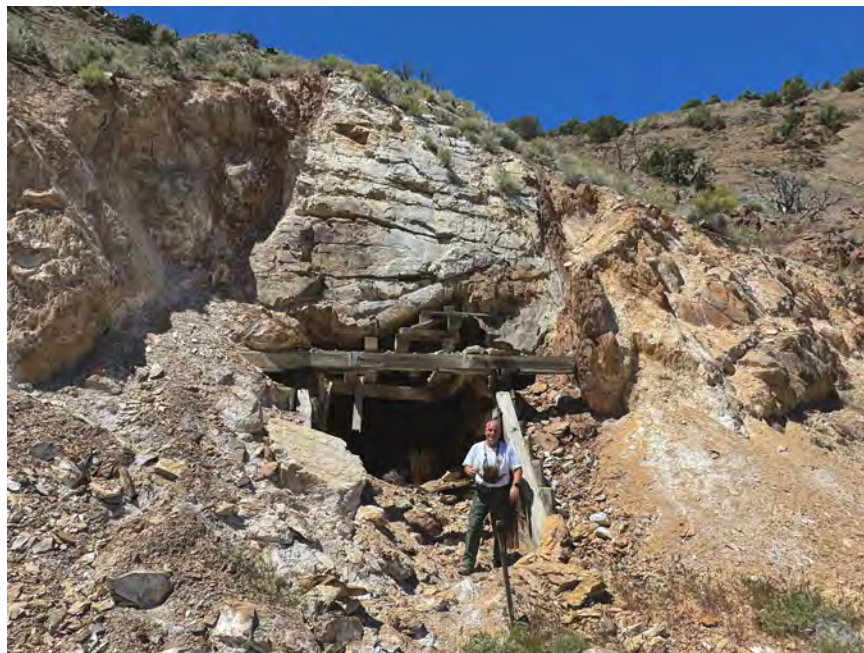
Figure 19: Entrance to the middle Arrance adit; note the latite dyke
