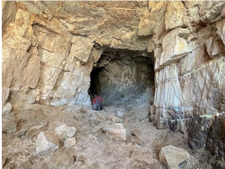
Figure 20: Middle Arrance adit, developed in the hydrothermally altered latite dyke hosting fracture-controlled mineralization
