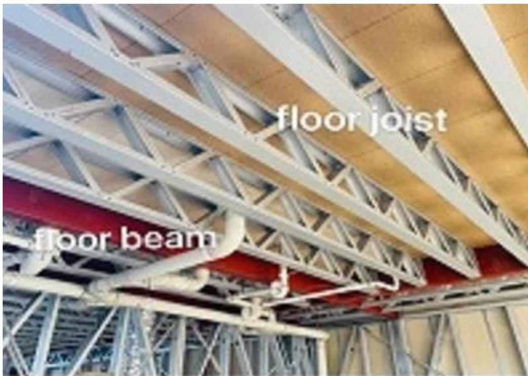
Figure 18. Construction site floor structure.
