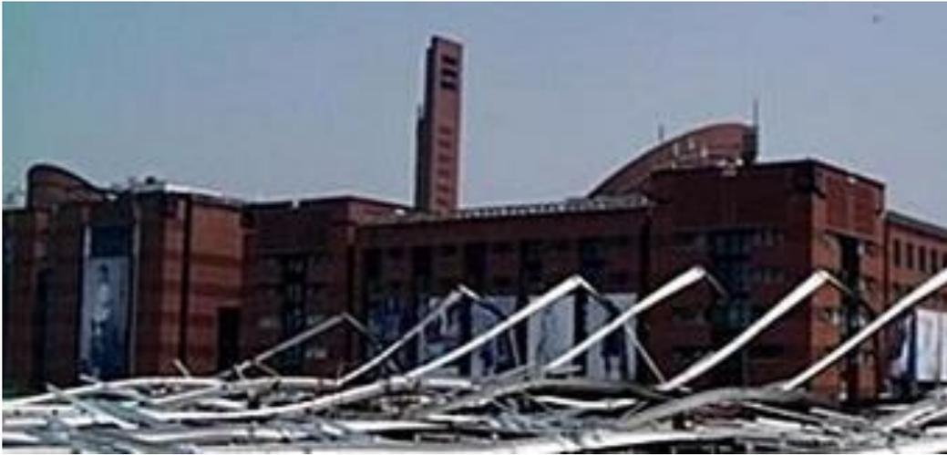
Figure 2. Collapse site of steel frame of factory building under construction (Wang, 2009).
