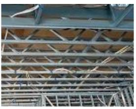
Figure 1. Site view of CFS joists
