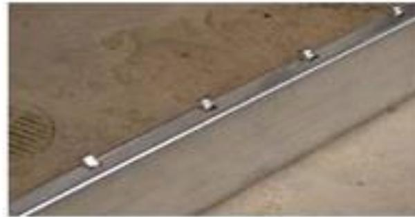
(b) Pre-fabricated bent-up tabs.
