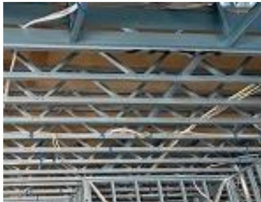
Figure 1. Site view of CFS joists
