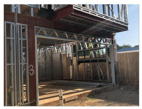
Figure 2. Frame and wall structures of a domestic building, by Huiyue Qiao.
