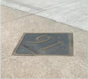
Pictured to the left is an example of a concrete-embedded formed metal, which can be manufactured to display the Village logo. The material is slip-resistant and could be installed in select high-traffic pedestrian and cyclist locations to create a unique impression for passersby.
