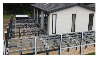
Liniar's steel sub-frames are designed for easy installation. The steel is pre-slotted so no pre-drilling is required and the PVCu sub-frame nogging is a quick and cost-effective way to connect all sub-frame joinsts with minimum preparation work.
