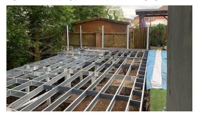
Liniar's sub-frame consists of only two components - the galvanised 'i' beam and the unique nogging connector. They are installed into a grid pattern and deckboards are fitted directly to the joists.
