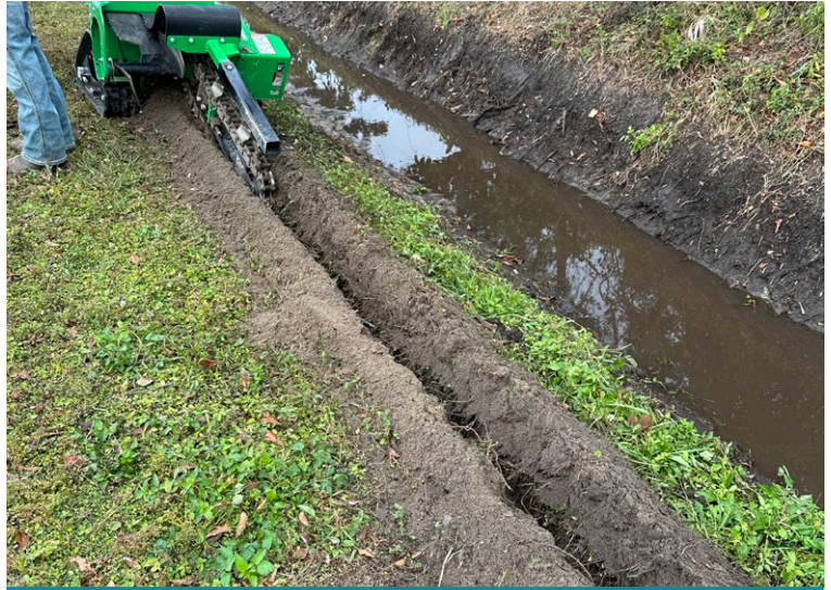
Ditch re-profiles with anchor trenches
