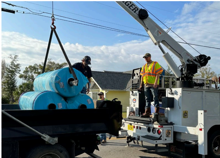
CCX-M™ Bulk Rolls unloaded using crane truck and spreader beam
