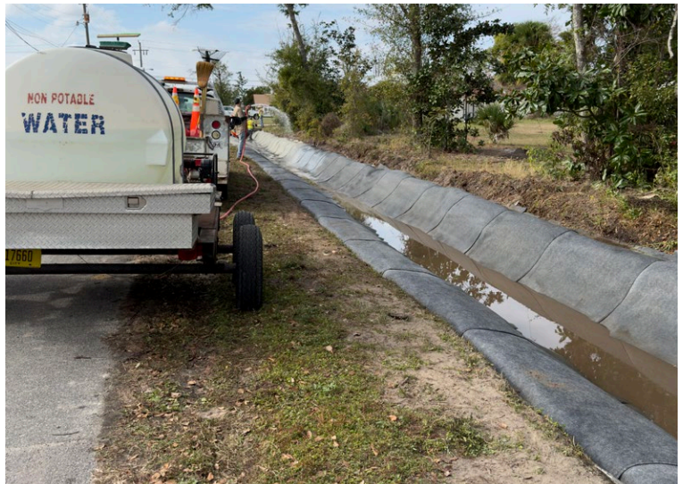
CCX-M™ Hydrated using a water trailer and hose
