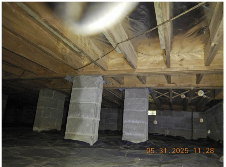
Damaged joist with new joist installed.
