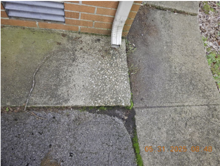
Discharge at foundation.
