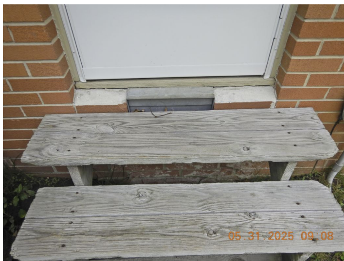
Moderate deterioration and protruding nail.
