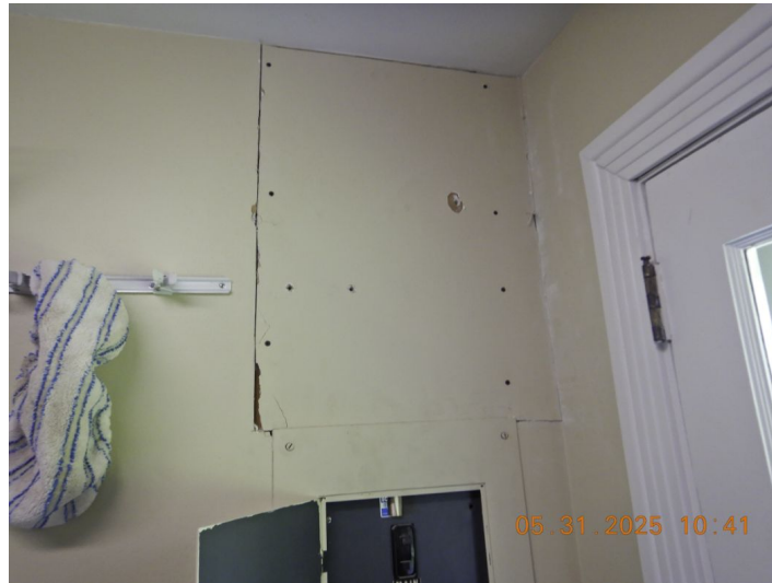
Likely wall cut to aid in electricla upgrades .
