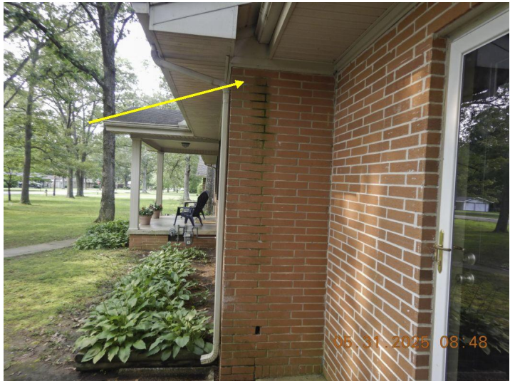
Overflowing or leaking gutter.
