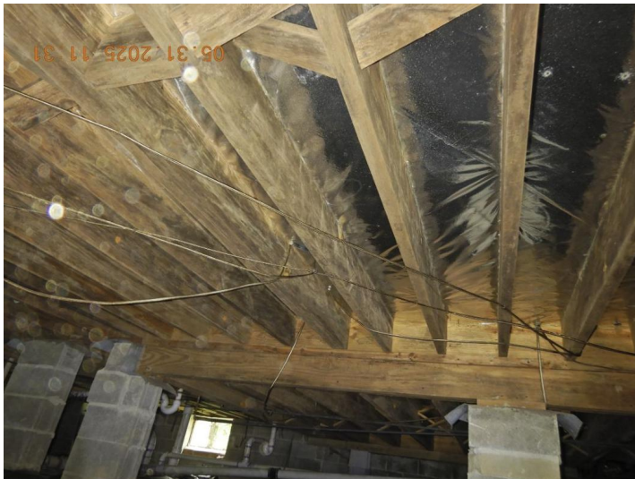
New joists sistered to olde (damaged) joists.
