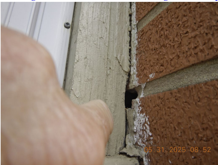
Damaged or missing caulking.
