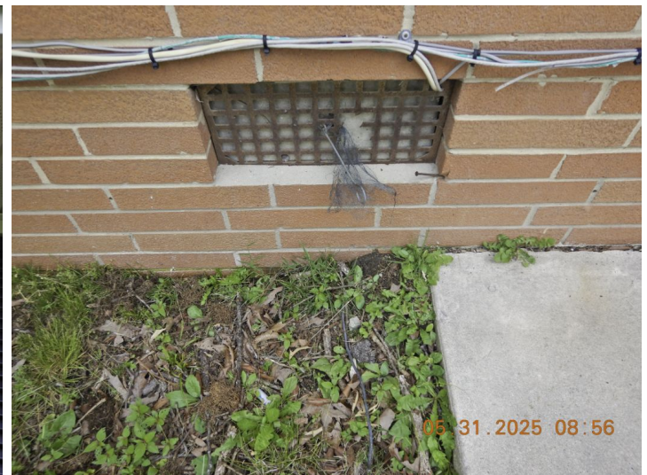
Damaged crawlspace vent.
