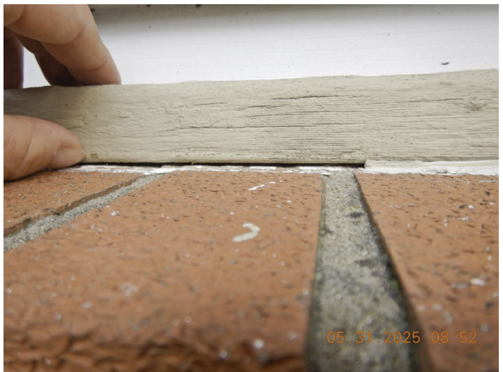
Damaged or missing caulking.
