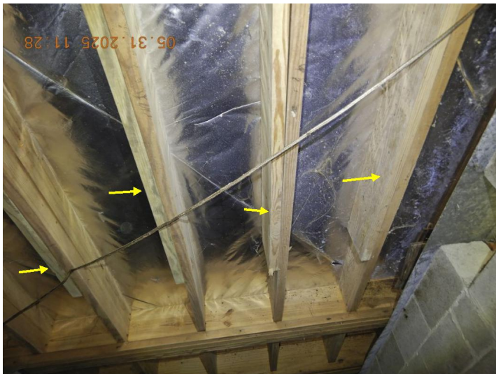
New joists sistered to olde (damaged) joists.
