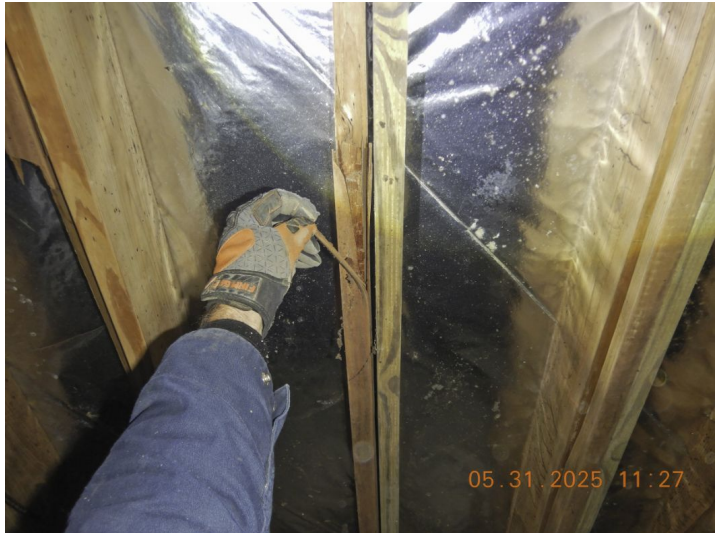
Damaged joist with new joist installed.
