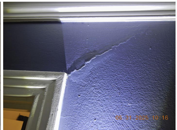
Small corner crack.
