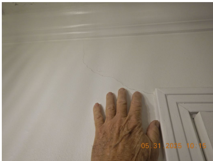
Small corner crack.
