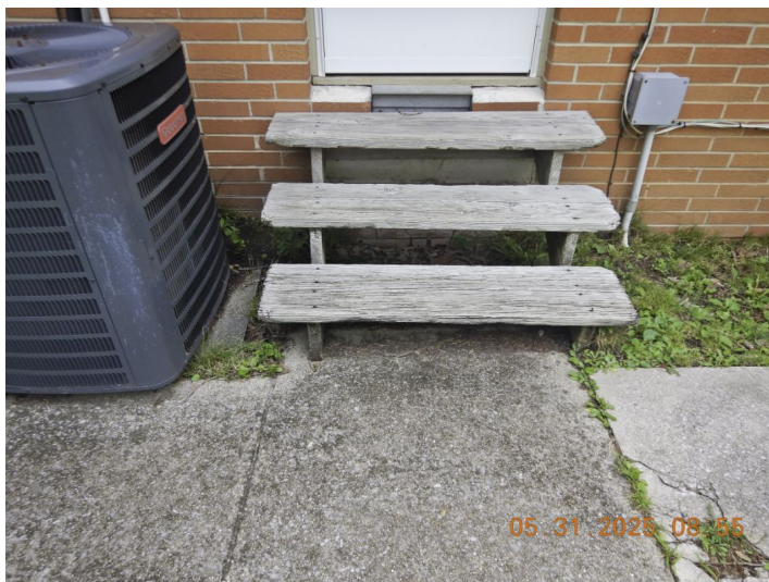
Moderate deterioration and protruding nail.
