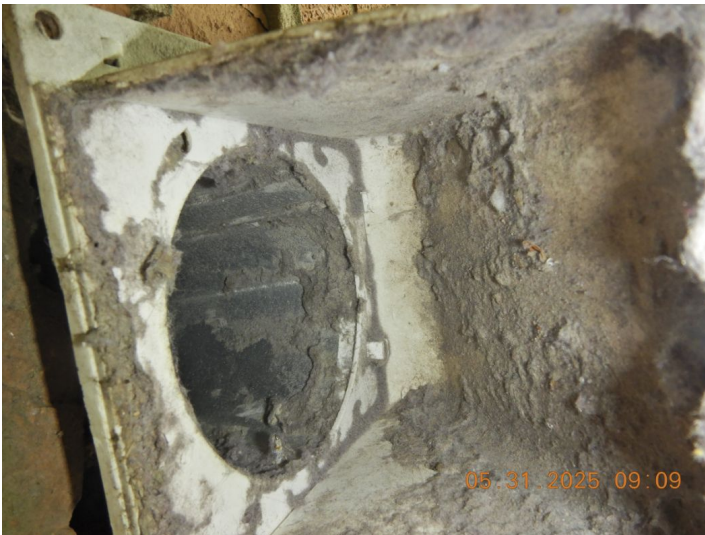
Clothes dryer vent missing flapper.
