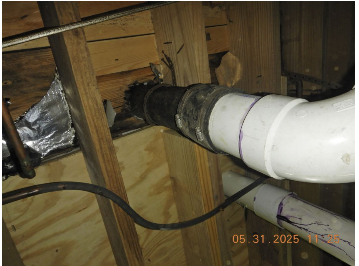
PVC and cast iron vent pipe.
