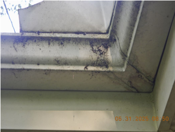
Overflowing gutter.
