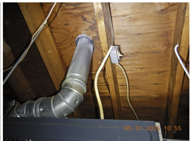
Junction box (switch) missing cover.
