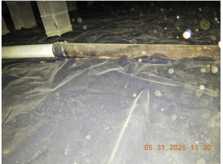
PVC and cast iron vent pipe.
