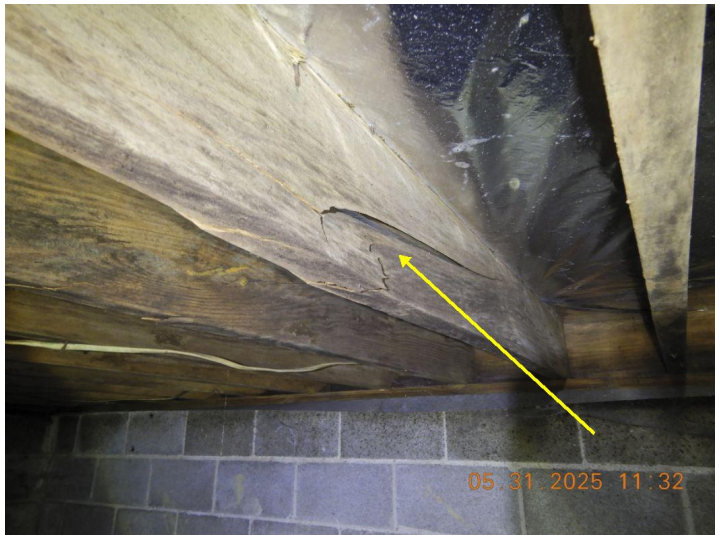
Damaged floor joist, needs repair.
