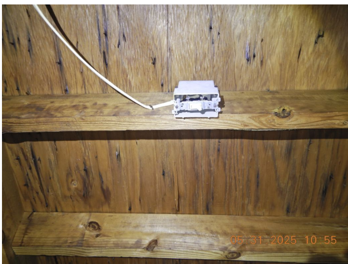
Junction box (switch missing cover.
