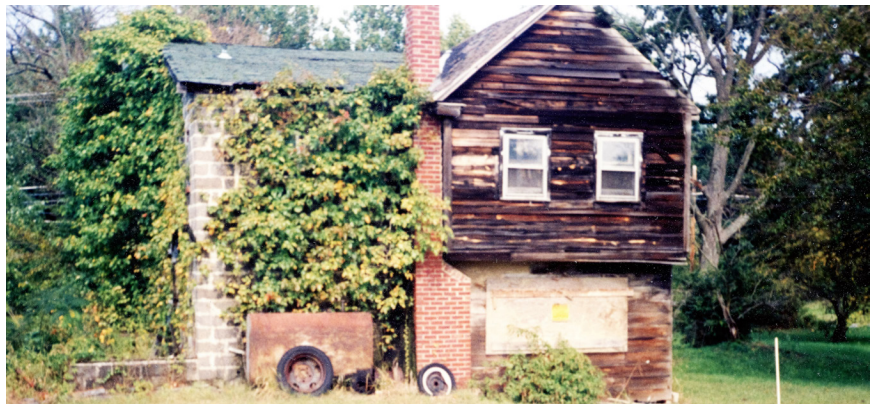
Figure 5 Former home of Major Mitchell and his descendants, demolished in 1996. Clapboard portion on the right is the original structure; left side cinderblock portion was added sometime after 1959.
