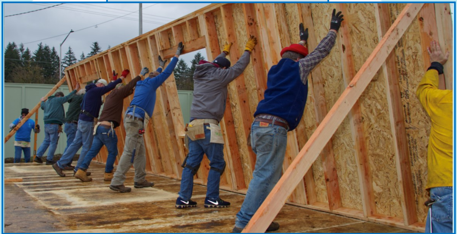
The guys putting one of the walls up!
