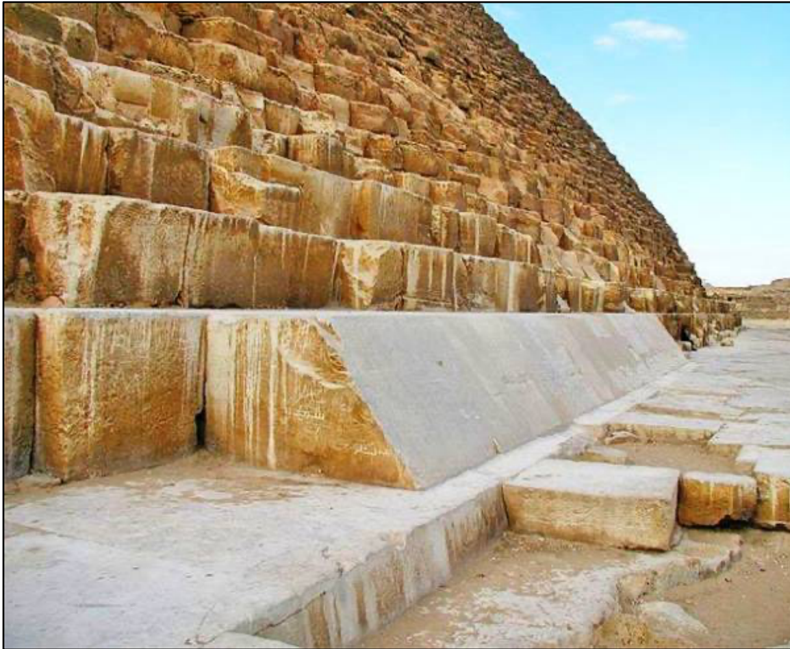
Figure 4. Polished White Casing Stones
