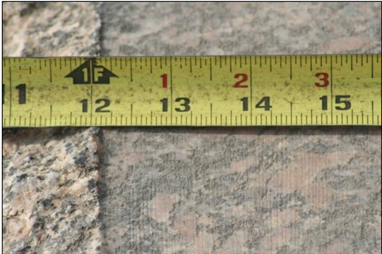
Figure 25. Machine Feed Marks
