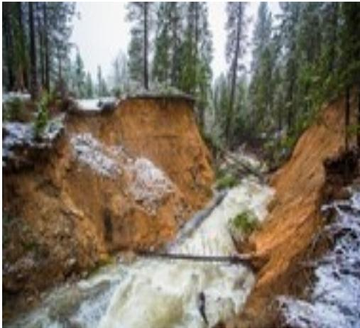
Fueled by an atmospheric river that funneled a vast amount of moisture into Northern California, the severe winter storms that hit last month caused countywide damage. Perhaps the most prominent is the culvert failure and washout of Morton Road in Alta. The incident isolated 15 homes (**and Camp Norge**). An alternative access was established, however it traverses a steep, windy gravel road over private property.” The picture above is where the road used to be and you can see the depth
