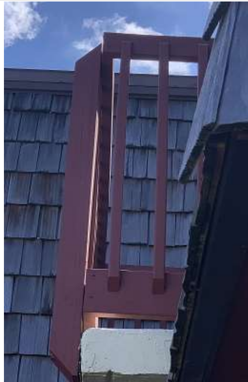
Balcony posts attached at the front of the stucco balcony slab
