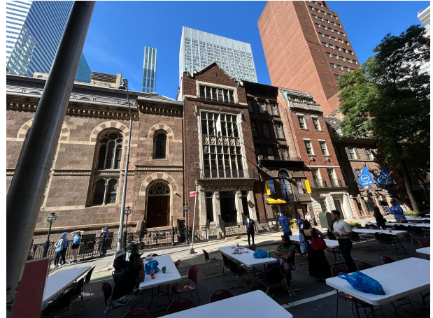
East 55th Street frontage. Photo by DB Landxpert LLC.
