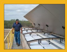
The AX-Mobile uses textile sheets in a packedbed media filter. It can treat blackwater and greywater to a level where effluent can be reused for surface or subsurface irrigation or for dust control (as regulations permit).
