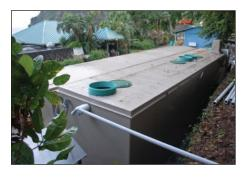
At only 7 ft (2.1 m) wide and 12,000 pounds (5443 kg), the units were trucked to the site down steep, narrow roads on the back of a standard flatbed and lifted with a crane. Less than two days after reaching the site, the system was up and running, in spite of power fluctuations and other challenges. An addition to the treatment system is currently in progress.
