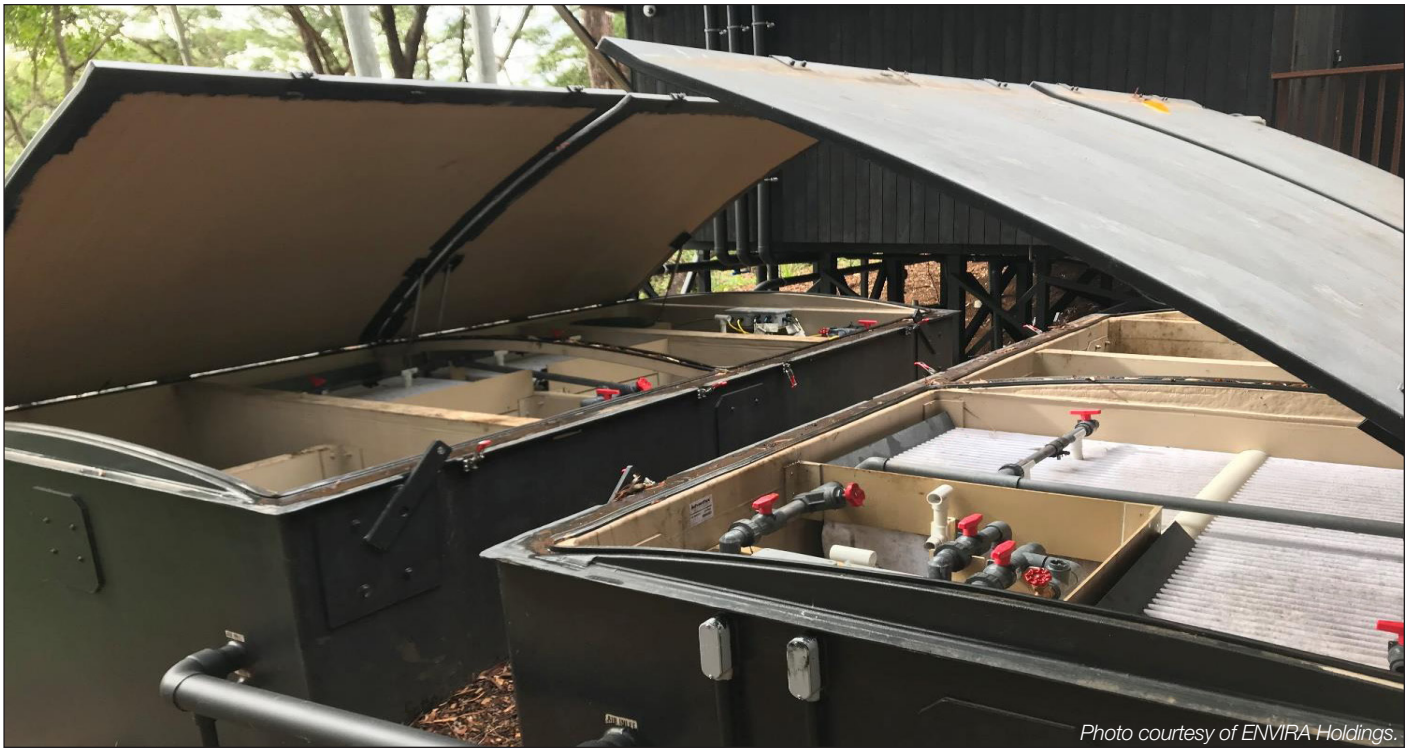
These AX-Max units were custom designed to work together at this campsite. Integrated into the unit on the right is an 8300-L (2200-gallon) tank that's divided in half to accommodate both primary and pre-anoxic chambers.
