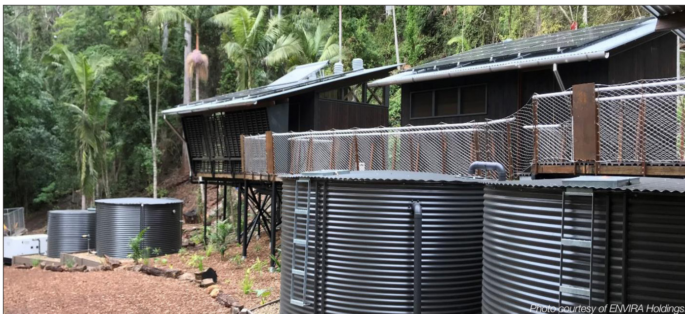
Treated effluent from the AdvanTex system is clean enough to be reused as subsurface irrigation. Left to right, the storage tanks at this off-grid camp contain treated AdvanTex effluent, rainwater for fighting bushfires, and rainwater that will be treated and used as potable water (two tanks).
