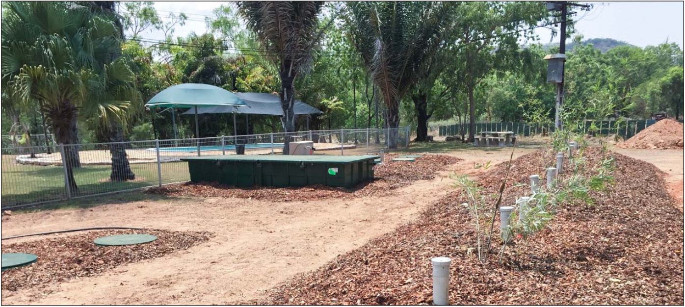
The AdvanTex AX100 Treatment System provides high-quality secondary wastewater treatment. Treated effluent is then dispersed through an ENVIRA Integrated Transpiration System (ITS®), consisting of evapotranspiration beds (shown above, on the right) planted with select vegetation.
