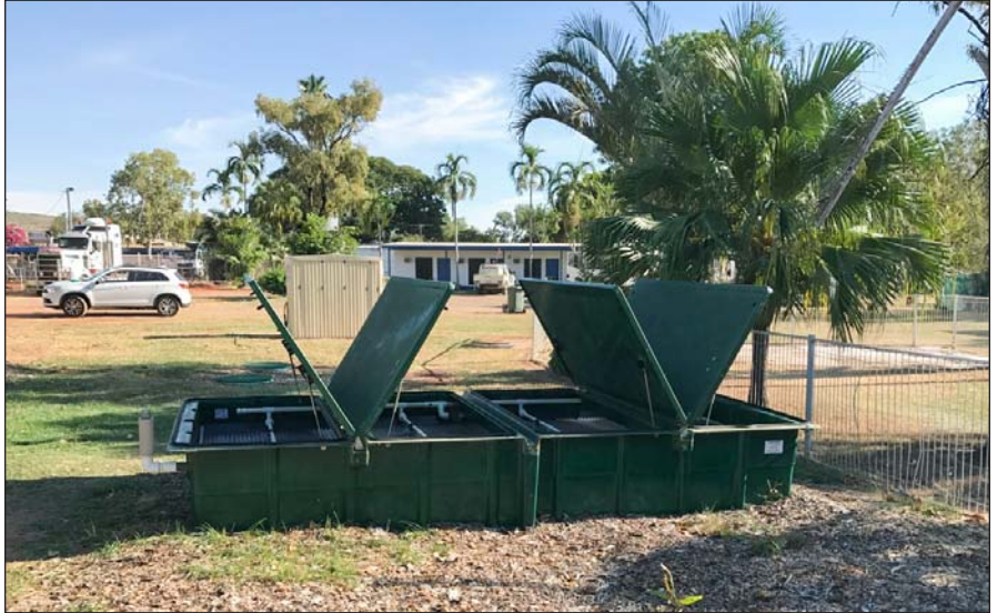
Because AdvanTex units can be installed in phases, the park will easily be able to expand its wastewater treatment capabilities in the future. Photo courtesy of ENVIRA Holdings.
