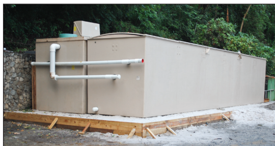
The resort needed two AX-Mobile units — one for tankage and one for treatment — to meet its emergency wastewater needs, and has since added two more treatment units. These will become part of the resort's permanent wastewater solution.
