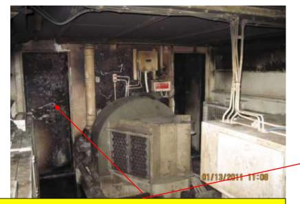
Operate the foam line from this door into the engine compartment.
