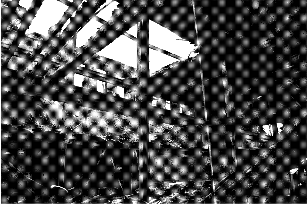
Figure 31 – Oxidized I-beams in the northeast corner facing southwest.
