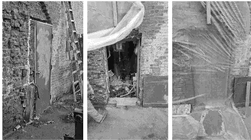
Figure 7 - Side by side pre-fire images of the north exterior metal door in place, the metal door removed, and the plywood and plastic sheeting.
