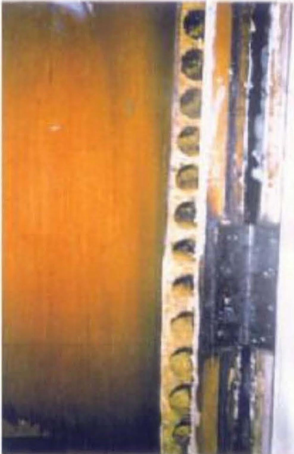
*Photograph No. 5 –A 'tube board' fire-resisting door with hollow tubes in the chipboard (fibreboard) inners*
