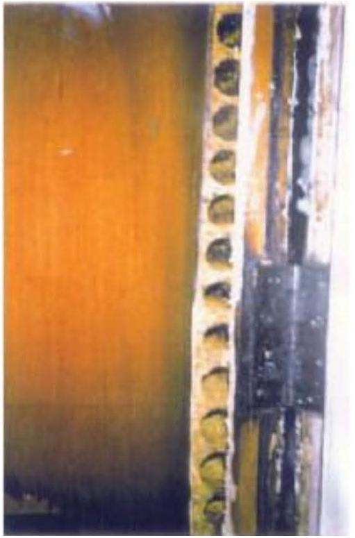
Photograph No. 5 – A 'tube board' fire-resisting door with hollow tubes in the chipboard (fibreboard) inners
