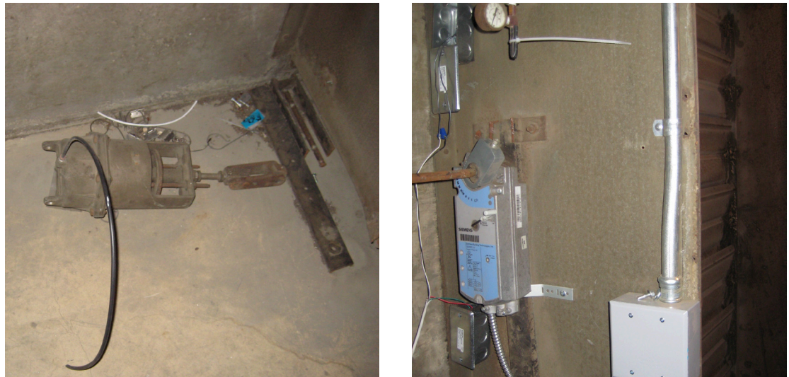
Figure 4-4: Photographic evidence showing replaced economizer damper actuator
