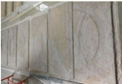
9. Leveling the pattern by net and sand
