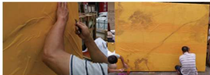
2. Removing the bubbles
