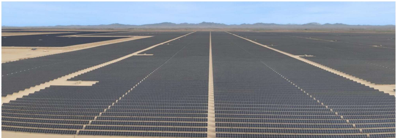
Desert Quartzite solar project, Blyth, California: 300 MW electricity generation, 150 MW storage. Project land requirements: 3,000 acres. Project Cost: $1 billion. Produces “clean energy” for up to 120,000 homes.
