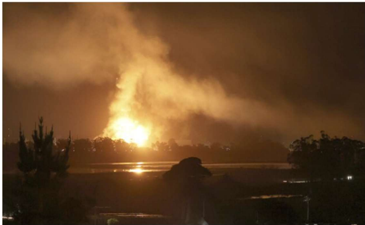
Moss Landing Energy Storage Facility Fire, January 16, 2025.
