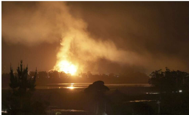
Moss Landing Energy Storage Facility Fire, January 16, 2025.
