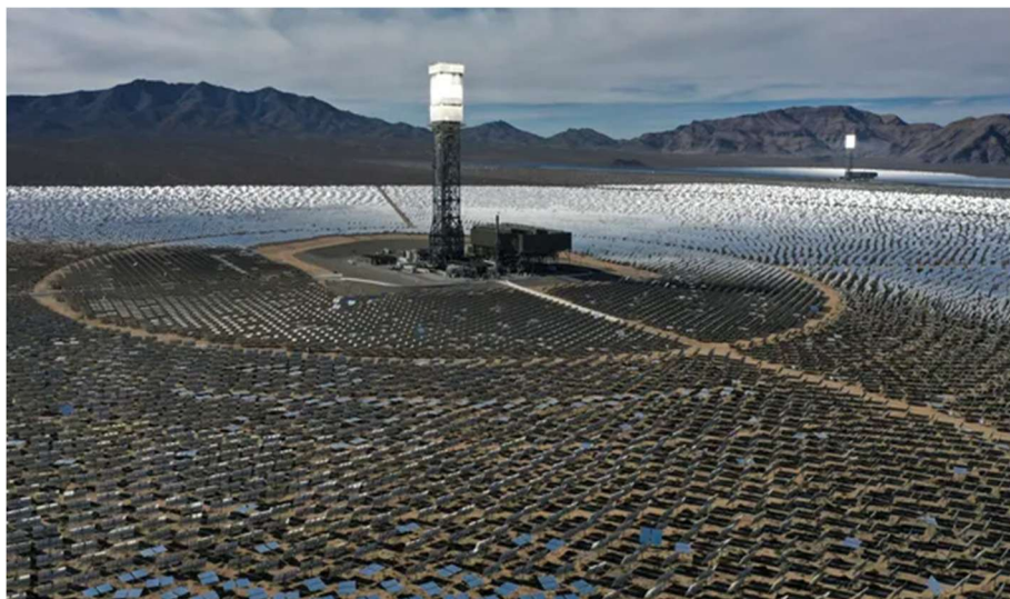
Ivanpah Solar Power Facility, San Bernadino county, California.
