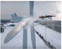
Note: Researchers have found that icing has a major effect on wind turbines. Even under high wind conditions, iced wind turbines have been found to rotate much slower and even shut down frequently during the icing event, with icing-induced power losses of up to 80%.
