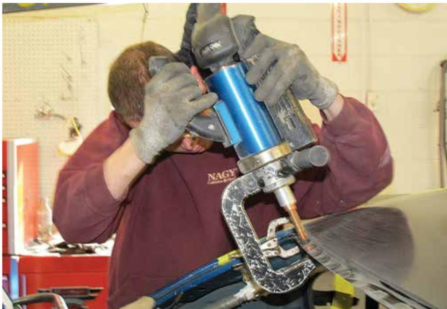
***This technician has access to both sides of the panel and thus can produce a structurally sound spot weld. But what happens when you cannot access both sides?***
