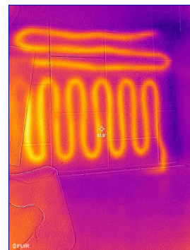
Radiant heat in the upstairs bathroom.
