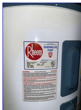
The Water Heater Data Tag
