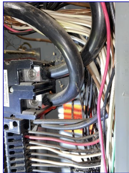
Aluminum Service Conductors
