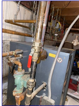
I observed corrosion on multiple parts of the boiler. The boiler worked fine. The boiler is past the normal operating life span. I recommend budgeting for a new boiler.
