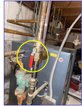
The Gas Valve Shut-off.
