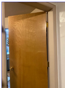
A photo of the garage door that needs an auto closure device added.
