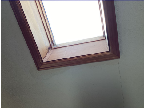
There were indications of moisture around the skylights. I recommend a licensed contractor evaluate and repair.
