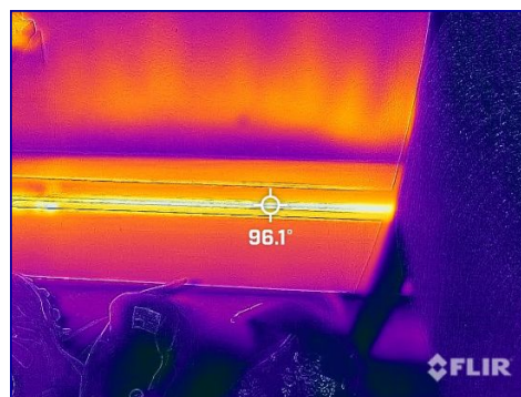
The boiler pumps hot water thru the system.
