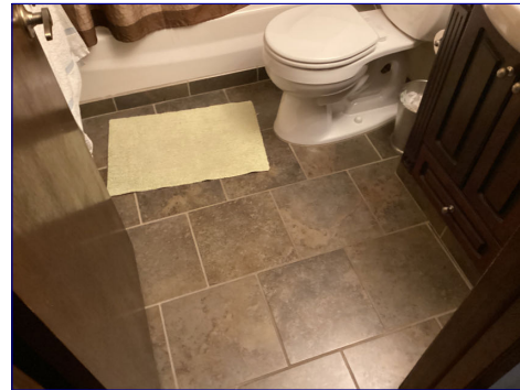
Electric in floor radiant heat in the upstairs bathroom.
