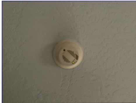
The yellow color of the smoke detector indicates old age. I recommend replacing the smoke detectors.
