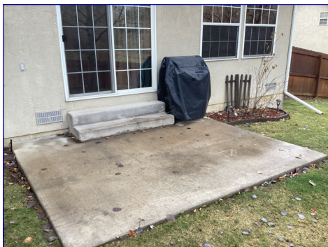
Because of the fact that there are uneven risers and multiple steps, I recommend the patio stairs should have a railing for safety reasons.
