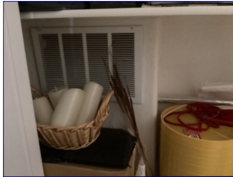
Access panel for radiant heat located in second-floor hallway closet.
