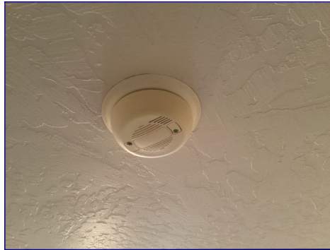
The yellow color of the smoke detector indicates old age. I recommend replacing the smoke detectors.
