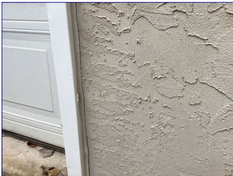
I recommend monitoring the caulking around windows, doors, corners, and utility penetrations to prevent moisture and pest intrusion.
