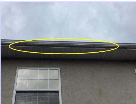
The fascia needs routine painting maintenance. I recommend a qualified professional paint the fascia.
