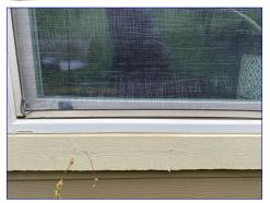
Some window screens are torn, damaged, or missing. Repair as needed.
