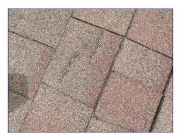
Roof covering showed signs of curling, cracking, and aging. I recommend a qualified roofing contractor evaluate and
