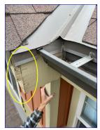
Gutter flashing was missing or insufficient. Adding gutter flashing will help direct the water into the gutter instead of allowing it onto the fascia. I recommend a professional roofer repair.
