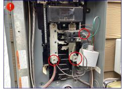
There are lugs double tapped with the surge protector and feeder cables and the white wire coming from the 25 amp breaker is hot and needs to be labeled. I recommend a qualified electrician evaluate and repair.
