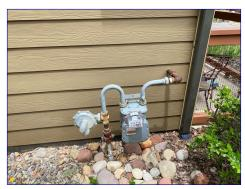
Gas service pipes show corrosion. I recommend contacting the gas provider to service equipment.
