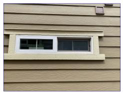
This window was installed upside down. The weep holes are at the top of the window frame in the photo. I recommend monitoring for water damage and repairing or replacing if needed.
