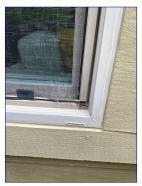
Some window screens are torn, damaged, or missing. Repair as needed.
