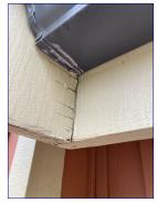
There is evidence that the gutter is leaking at the seams. I recommend a professional contractor evaluate and repair as needed.
