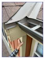
There are a few places on the fascia above the garage that are seeing water damage. I recommend routine painting maintenance. I recommend consultation with a qualified roofing contractor to discuss flashing options to prevent the water damage.
