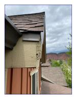
Adding flashing would help protect the fascia from moisture damage. I recommend a qualified professional repair.
