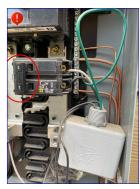
The AC unit requires a minimum circuit amperage of 27.6. The breaker for the AC unit is rated at 25 amps. I recommend a qualified electrician
