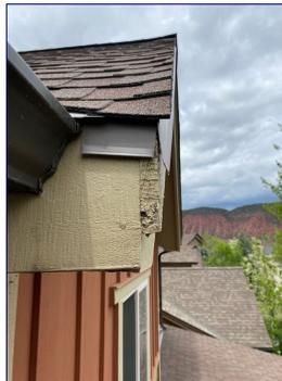
Adding flashing would help protect the fascia from moisture damage. I recommend a qualified professional repair.
