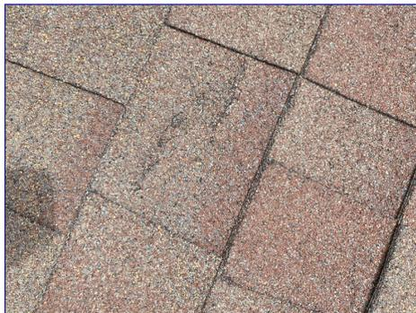
Roof covering showed signs of curling, cracking, and aging. I recommend a qualified roofing contractor evaluate and repair.
