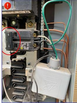
The AC unit requires a minimum circuit amperage of 27.6. The breaker for the AC unit is rated at 25 amps. I recommend a qualified electrician evaluate and make repairs.
