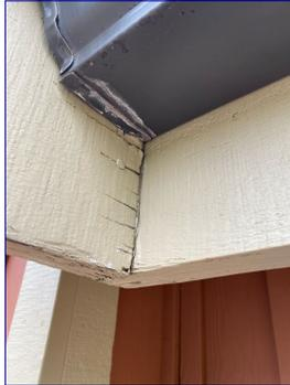
There is evidence that the gutter is leaking at the seams. I recommend a professional contractor evaluate and repair as needed.
