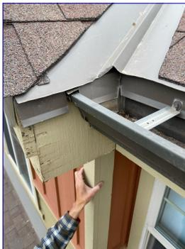
There are a few places on the fascia above the garage that are seeing water damage. I recommend routine painting maintenance. I recommend consultation with a qualified roofing contractor to discuss flashing options to prevent the water damage.
