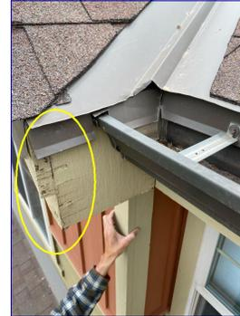
Gutter flashing was missing or insufficient. Adding gutter flashing will help direct the water into the gutter instead of allowing it onto the fascia. I recommend a professional roofer repair.
