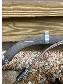
There is damaged and/or missing insulation on the air conditioner refrigerant line. I recommend replacing the insulation.
