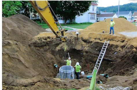
Water and Sewer Project in Prairie du Chien
