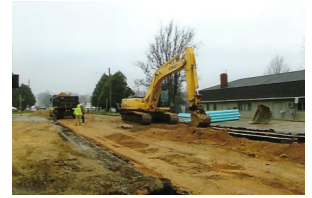
Waterline Extension to New Grocery Store in Fennimore
