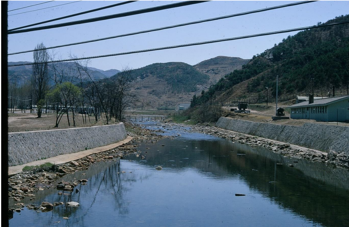
Monsoon drainage ditch, Camp Casey
