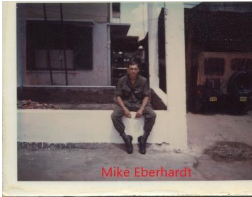
Mike sitting on what remained of their storage room located beneath the tower of the compound where MAT IV-5 lived. Their dwelling was in front of the jeep. The jeep belonged to the District Chief.
