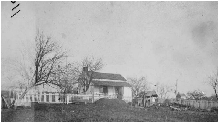
Meade's headquarters showing damage from Confederate cannons, with horse grave in front.
