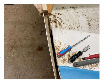
After removing all the remaining wood from the fiberglass transom by hand-scraping with a chisel, I sanded the back fiberglass panel using a 5" orbital sander with 60 grit sandpaper to get the last bits of wood off. In this photo, I had just finished the port side of the transom and was moving over to the starboard.
