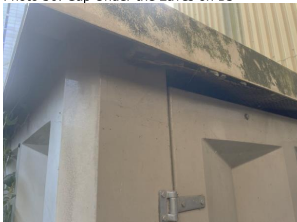
Photo 36: Gap Under the Eaves on B3
