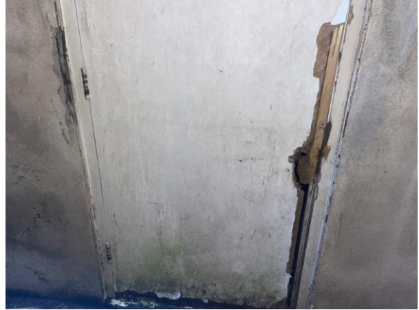
Photo 28: Interior of B2 Facing North, Gap in Brickwork
