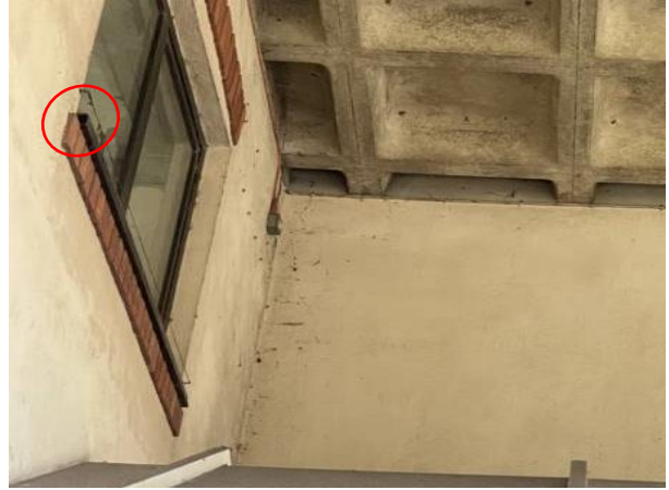
Photo 45: Exposed Corrugated Sheetting and Gaps in Brick Work in the Roof Access Point of B1b
