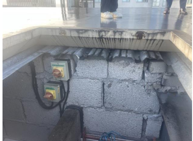
Photo 45: Exposed Corrugated Sheetting and Gaps in Brick Work in the Roof Access Point of B1b
