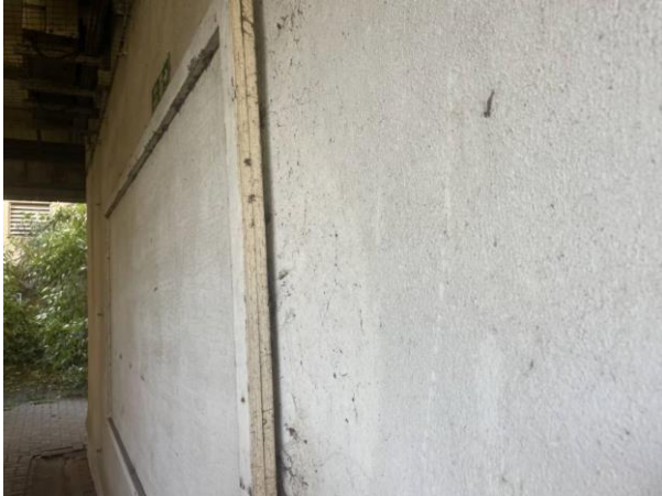
Photo 44: Gap in Rendering Underneath the Security Light to the Eastern Side of B1a
