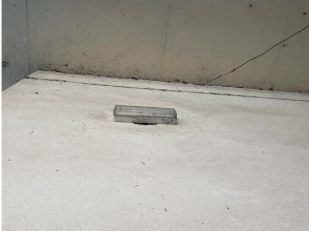
Photo 44: Gap in Rendering Underneath the Security Light to the Eastern Side of B1a
