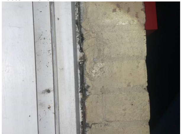
Photo 49: Gaps Surrounding Door Frame on the Eastern Front of B2
