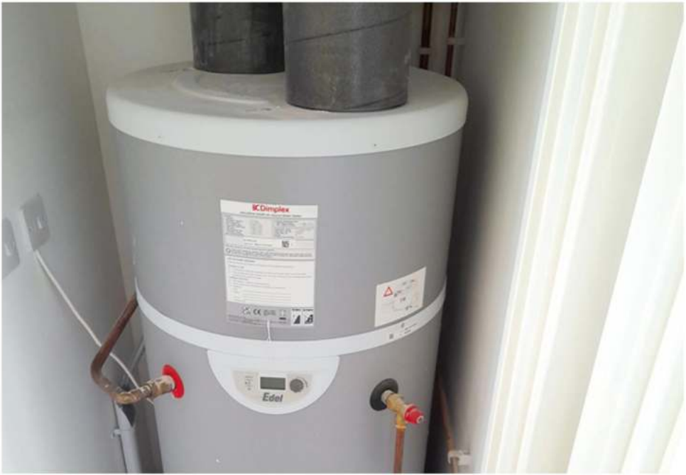
Unvented air source heat pump hot water cylinder
